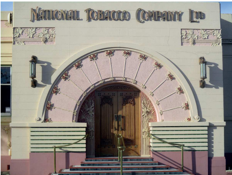
The National Tobacco Company Building in Napier.
